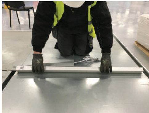
Seperate gear enclosure and insert Luminaire into noggin
