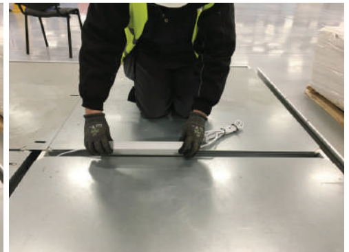
Carefully insert gear encloser into noggin
